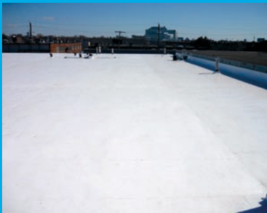
Toronto roofing contractor Guycan Aluminum installed 130,000 sf of single-ply roofing at Olympia Tile & Stone, Toronto, in the middle of the Canadian winter.
