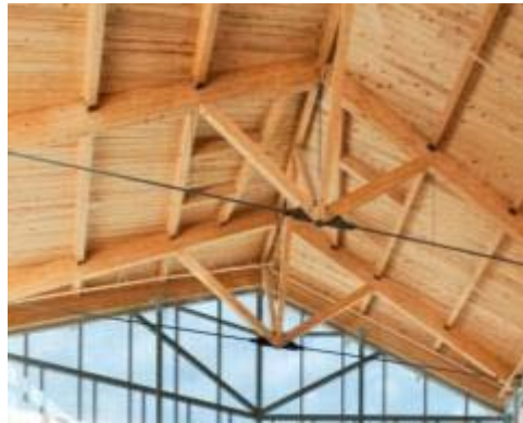
Student Center :: Roof Structure
