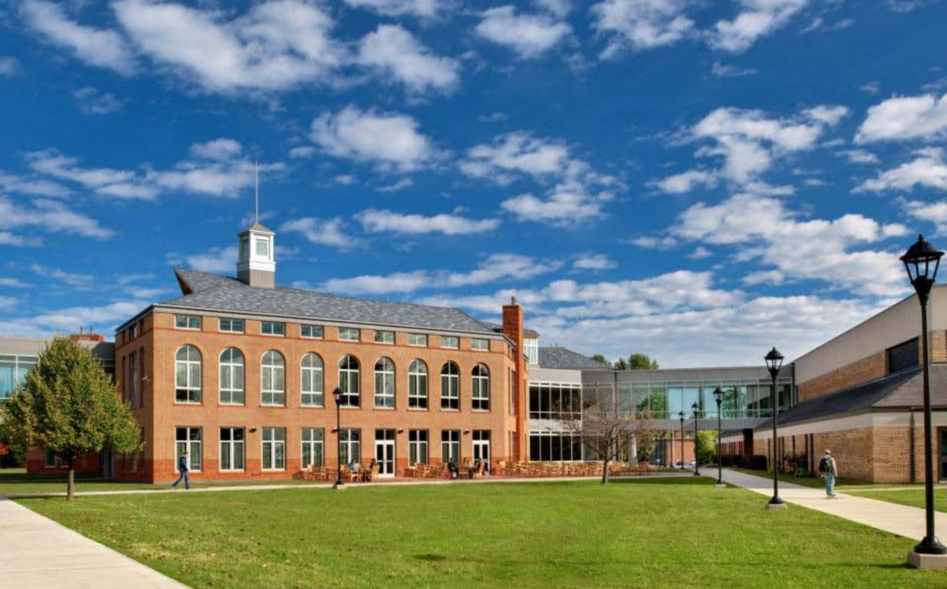
View of the Student Center South Façade
