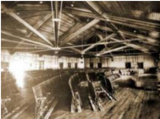
"Old Main" :: Roof Structure
