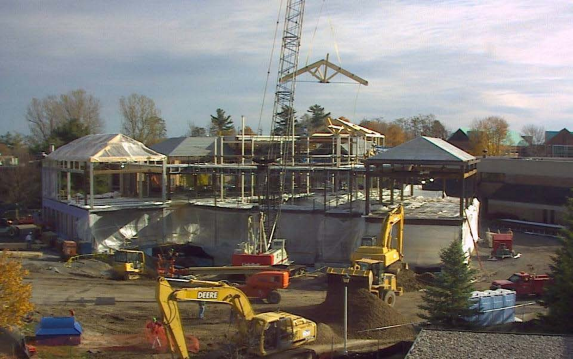
The dramatic wood trusses were manufactured off-site, and placed with a crane.
